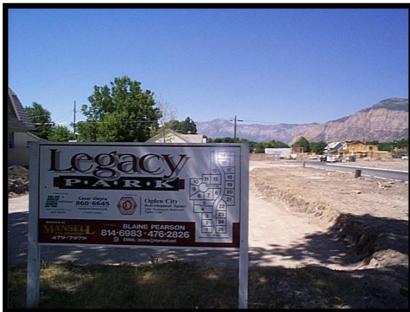
Figure 7.3 - Construction on the Legacy Park subdivision on 24 th Street
