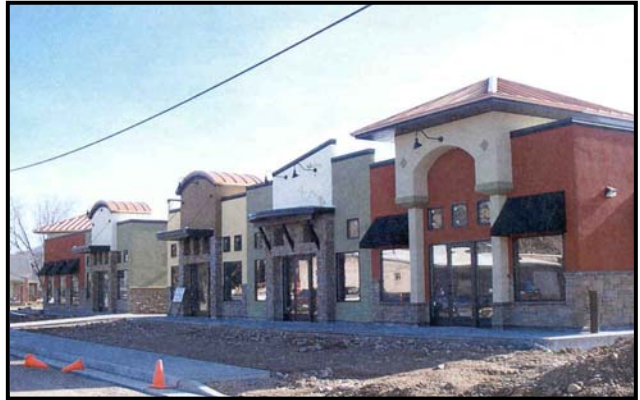
Picture # 3 – An example of building design; using different materials, roof styles and having the building façade fluctuate.
