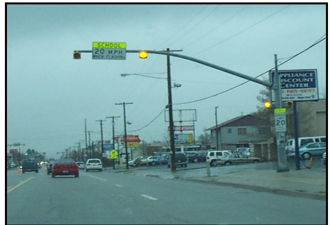
Picture # 8 – This is an example of a school crossing light that project out into the street.
